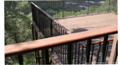
Deck with metal joist
